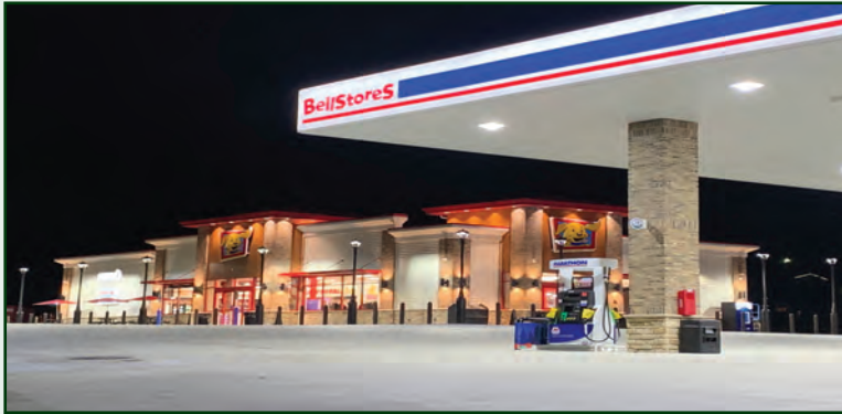
Photo above: New BellStores in St. Clairsville, OH, courtesy of Campbell Oil
