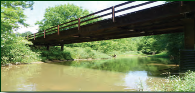
Photo shown above: Monroe County T307 Bridge
