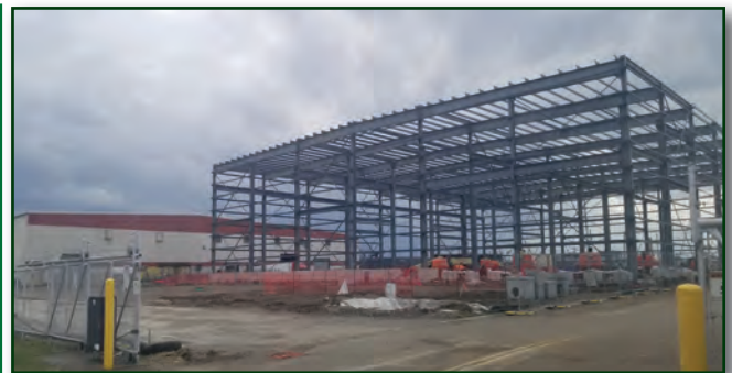
Photo shown above: New Ambaflex Operations Building under construction
