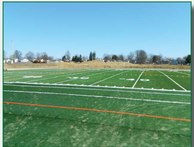
Photo above: New Massillon Track and Field, under construction in March 2018
