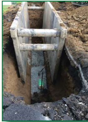
Photo above: Sanitary sewer trench box
