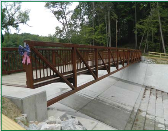
Photo above: New bridge and spillway at Camp Y-Noah
